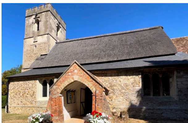
Thatched roof of All Saints, Rampton
